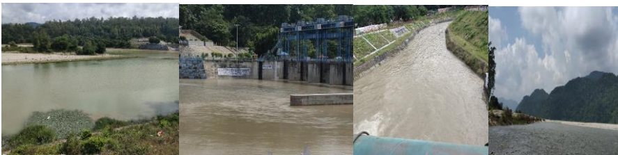
Source:- During Field Work Kosi Barrage 5 th October, 2022
